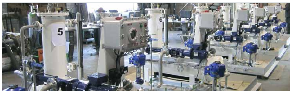
Dewatering packages under construction, with CVA actuators installed.
