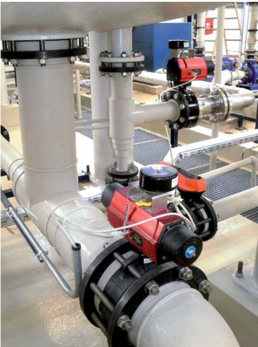
RC200 actuators at Sisak Power Plant, south of Zagreb in Croatia
