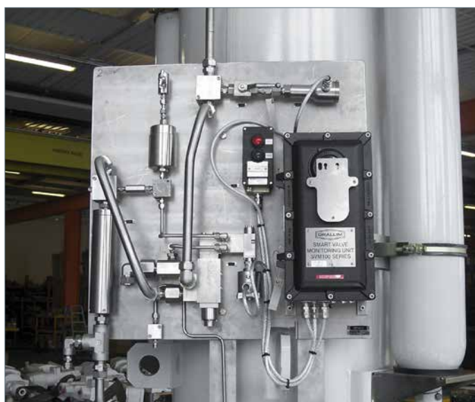
The Rotork SVM field unit is incorporated on the valve actuator control panel for hazardous area applications.
