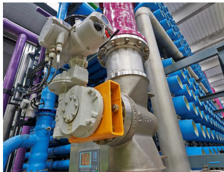
IQ actuator with IW gearbox at a water treatment plant in Spain
