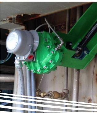
or instrumentation problem from the control room. Those symptoms contribute to a false read in the DCS. Some of the register dampers believed to have a damper drive problem were in fact frozen in place. Addressing both the damper bearings and the damper drives at the same time is very beneficial to ageing boilers.
