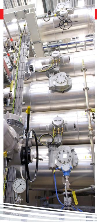
Safety is of primary importance and for this reason virtually all the ball valve installations are of double block and bleed design, the largest weighing in at eight tonnes. Security against leakage is vital for the accuracy of the metrology as well as safety.
