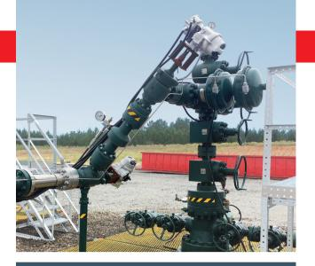
The lightweight, compact IQTF actuator provides fast and accurate valve control and can perform up to 1,800 starts per hour, an important factor given the need for a tight well flow threshold to avoid over pressure in the main trunkline.
