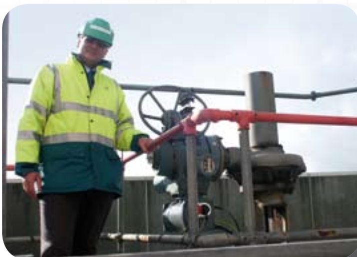
Rotork A range actuator with newly upgraded internal Pakscan field card at the BP terminal at Hamble.
