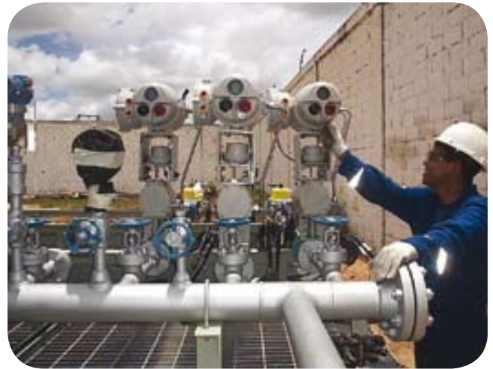
Above: Rotork Skilmatic SI actuators on a pipeline metering skid in Venezuela. Below: Skilmatic SI size 1 and 2 Linear and Quarter-turn actuators
