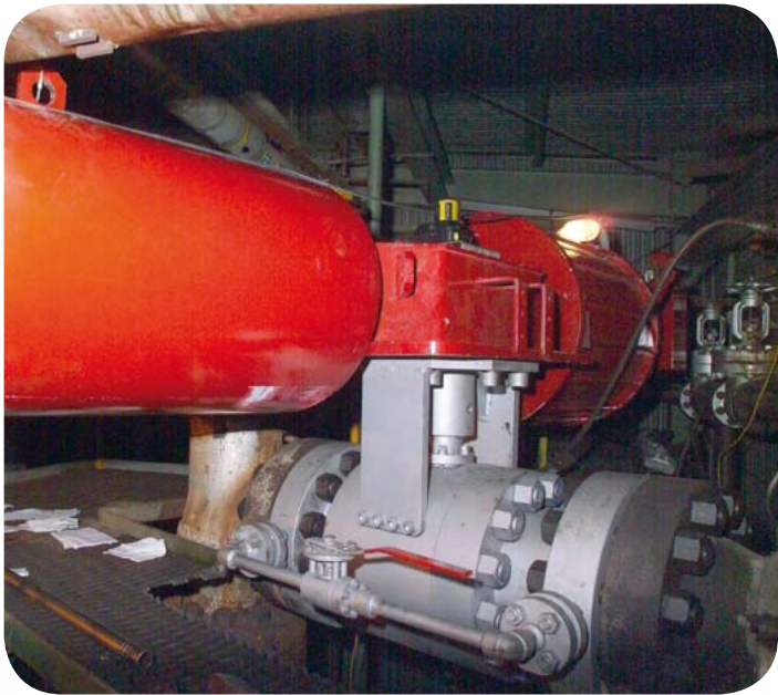
GP200 pneumatic, spring return actuator (model no. GP-200S-685/C2-HPA).
