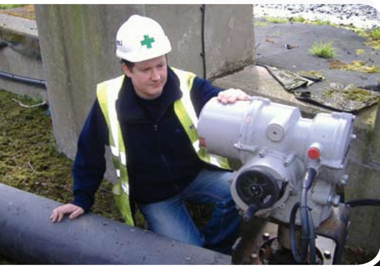
Above: Stuart Goodwill from Mott McDonald Bentley is pictured with one of the Rotork IQT actuators at Esholt.
