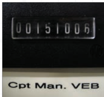
Counter fitted during the installation
