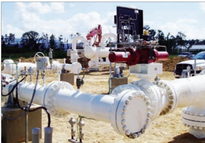
This specialised Rotork Fluid Systems HPG direct high pressure gas actuator provides vital over-pressure protection on a section of the Enbridge Pipeline in Canada
