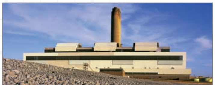
Aberthaw Power Station
