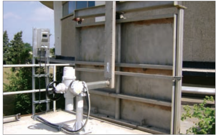
The finished actuated installation
