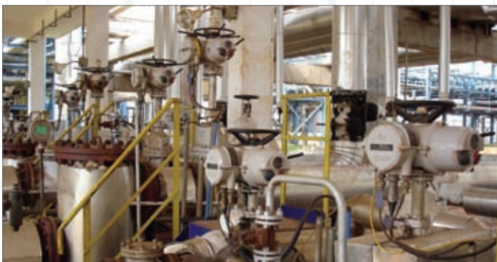
Rotork IQ Pro valve actuators installed on a processing area of the Qinzhou Refinery.
