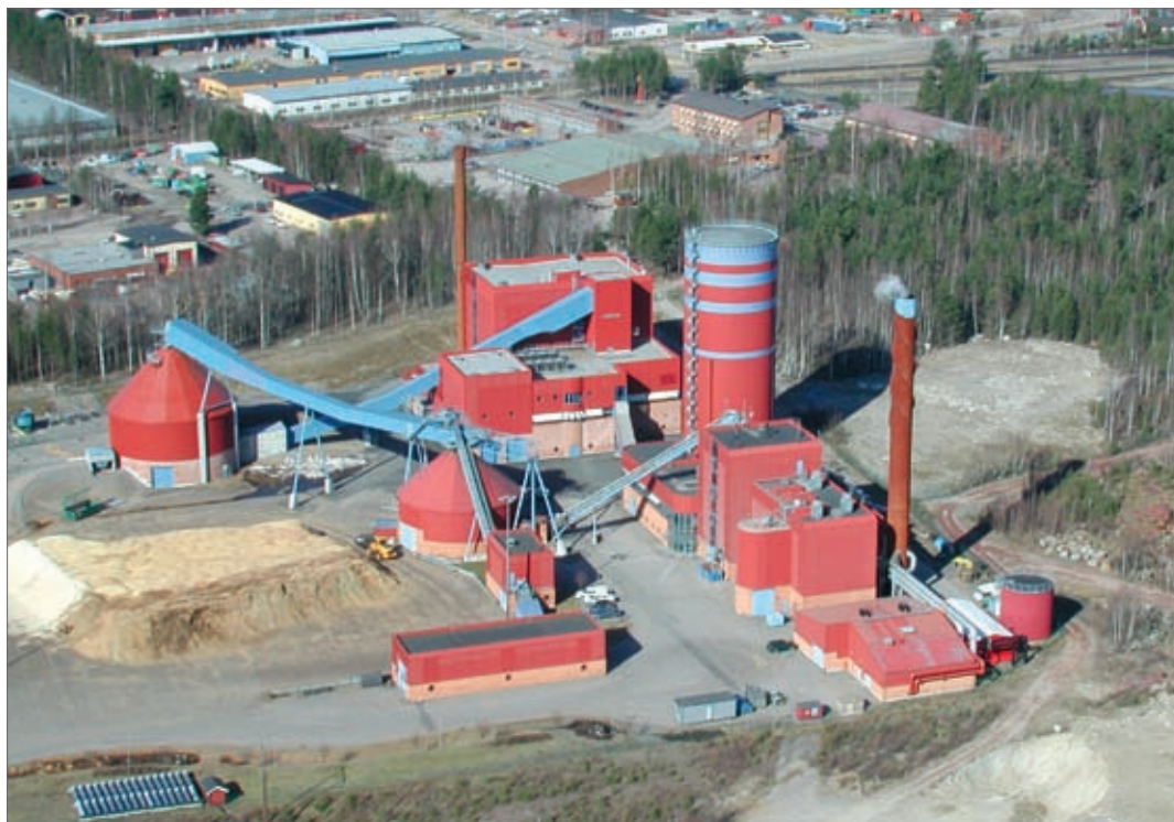
The Falun plant uses the latest Metso Hybex boilers with BFB (Bubbling Fluidising Bed) technology.
