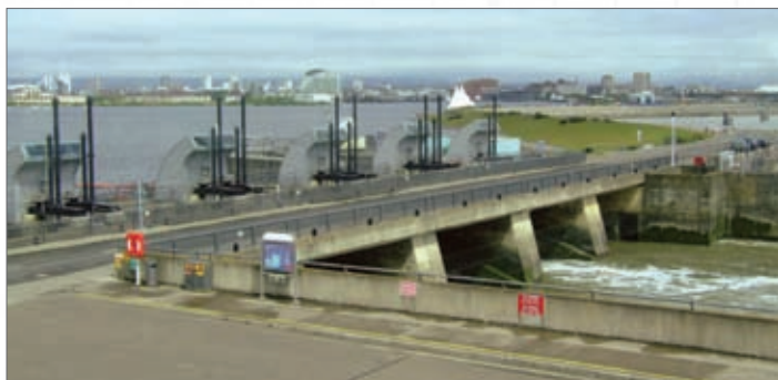
From the other side of the Barrage Control Room the five sluices that regulate the water level in Cardiff Bay can be seen, with the fishpass beyond and the bay in the background.
