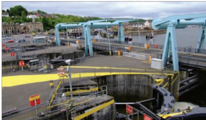
The landward view of the sea locks from the Barrage Control Room.
