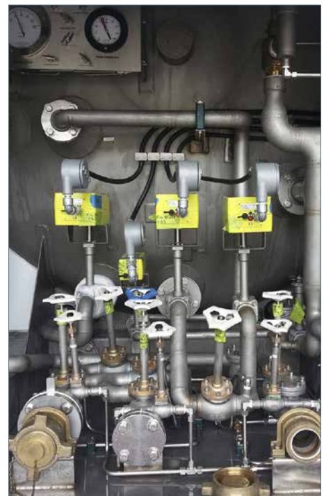
The Rotork Schischek ExMax actuator is successfully used in LNG cryogenic applications.
