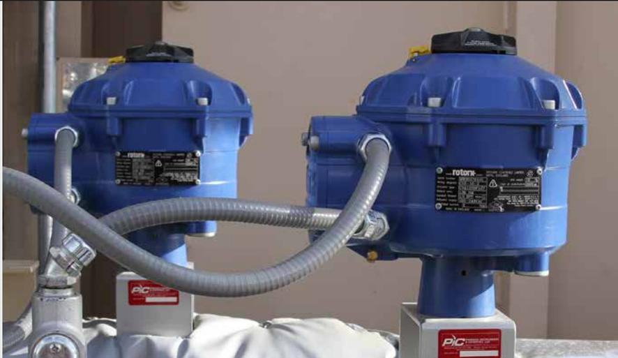
*Fig 3 – Rotork CVA electric actuators like this are used on separator skids, often as part of a solar energy package.*
