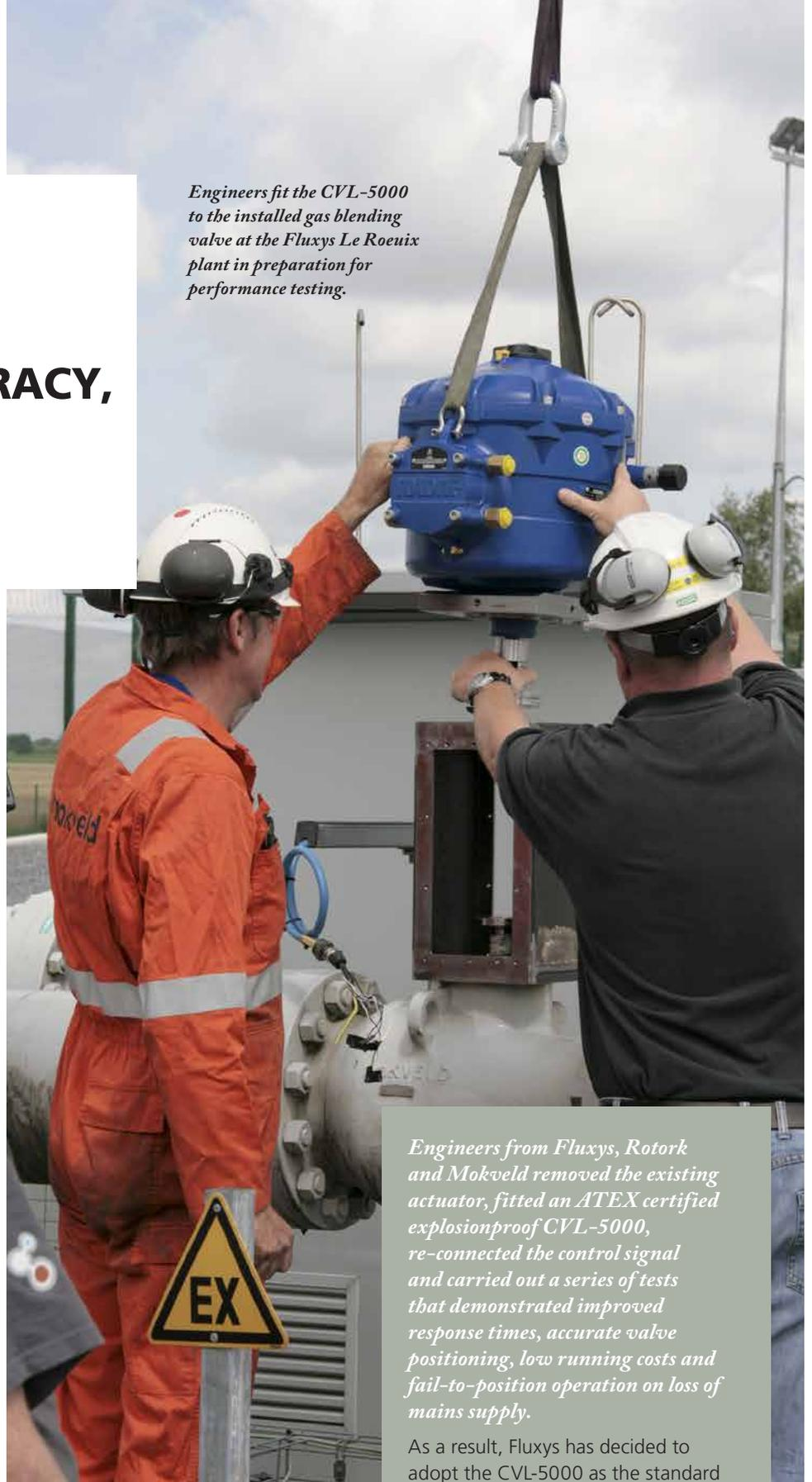
*Engineers from Fluxys, Rotork and Mokveld removed the existing actuator, fitted an ATEX certified explosionproof CVL-5000, re-connected the control signal and carried out a series of tests that demonstrated improved response times, accurate valve positioning, low running costs and fail-to-position operation on loss of mains supply.*
