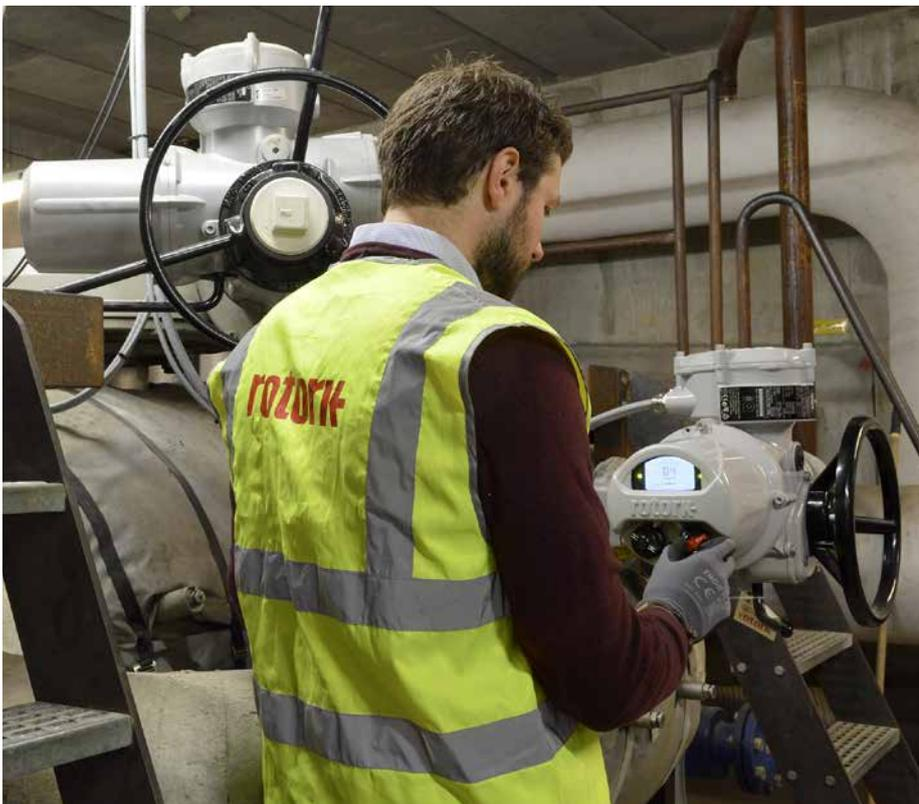
*Fig 2: A Rotork engineer inspects IQ actuators in another area of the valve chamber. The actuator at the top survived the immersion in near-boiling water; the actuator below has replaced one from another manufacturer that was permanently damaged by the flooding.*
