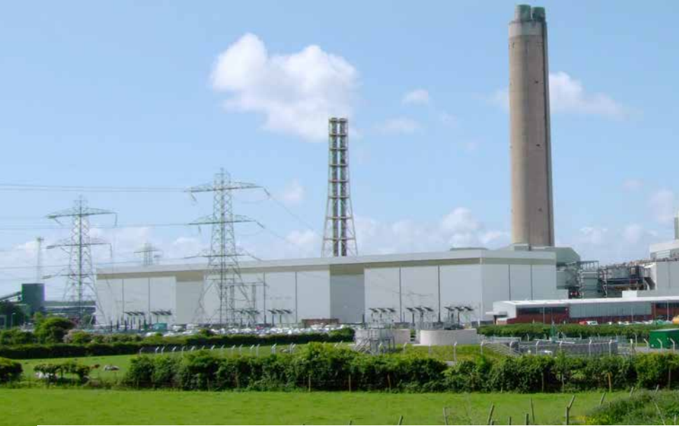
Aberthaw Power Station.
