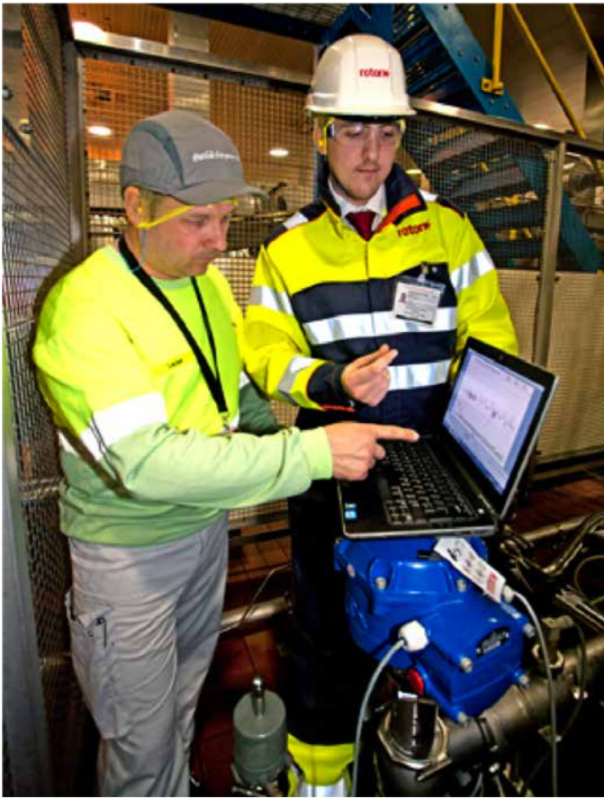
Installation and configuration of CVA actuator.
