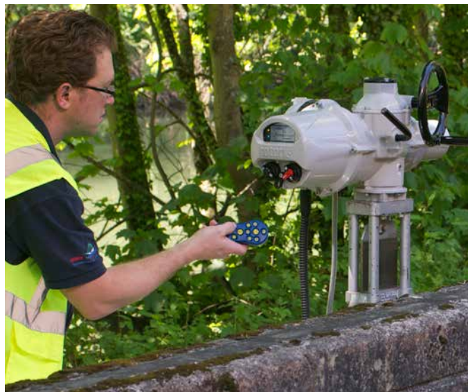
Wireless two-way communication using the non-intrusive hand-held setting tool is one of the secure means of accessing the asset management data in Rotork actuators.
