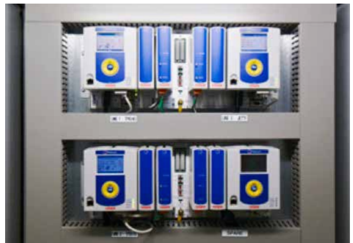
Pakscan Master Stations monitoring and controlling the IQ and Skilmatic SI actuators at BTT on three separate bus networks. Designed specifically for the valve actuation environment, Pakscan incorporates secure field communications with inbuilt network redundancy to maintain control even in the event of equipment or cable failure.
