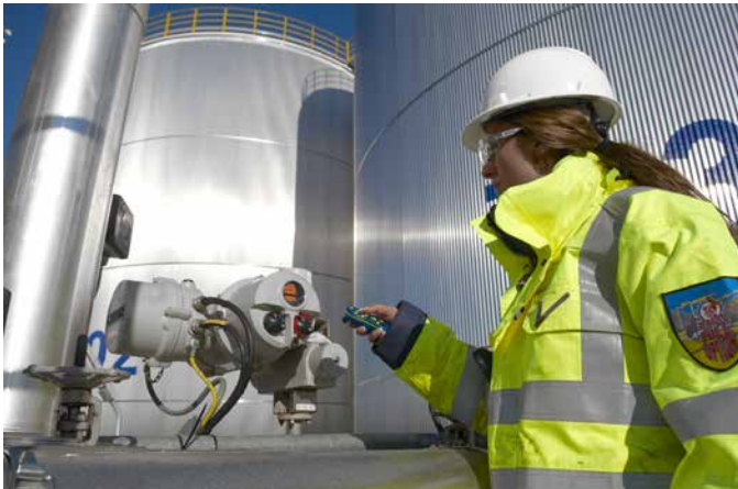
A non-intrusive, handheld setting tool is used to programme and commission the Rotork actuators, as well as download diagnostic information stored in data loggers.
