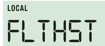
Fig 9.1 Fault history menu
