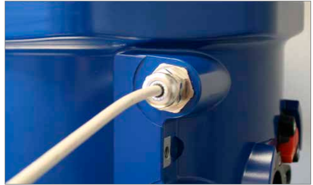
Fig 6.8 Cable gland installation
