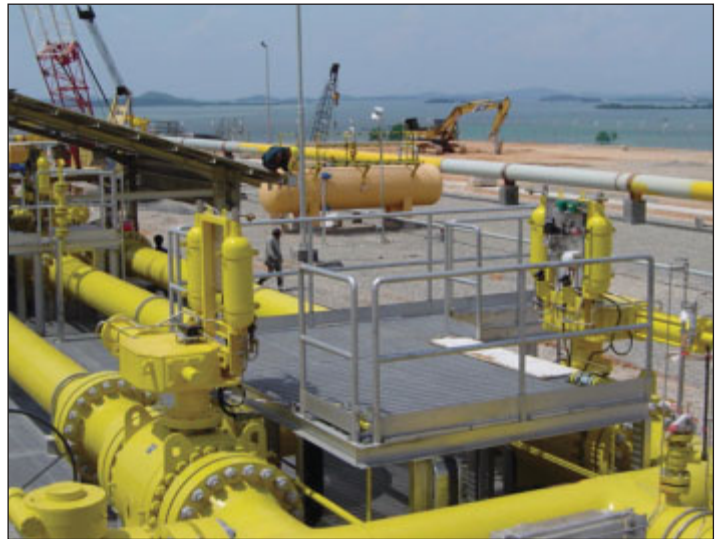
Right: Fluid system gas-over-oil actuators operating PBVS trunnion mounted ball valves (900mm) on skid mounted gas station metering duties.
