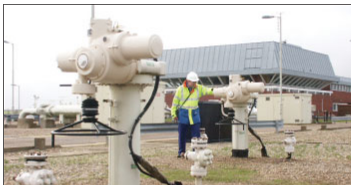
Pictured – new Rotork IQ70 actuators installed at NGT Bacton.
