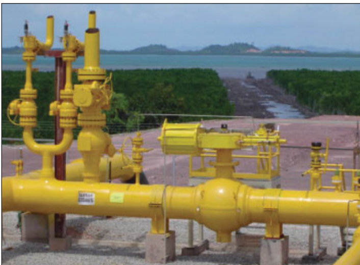
Below: Fluid System pneumatic actuator fitted to fully welded Cameron ball valve (900mm), providing gas station shut-off duty.
