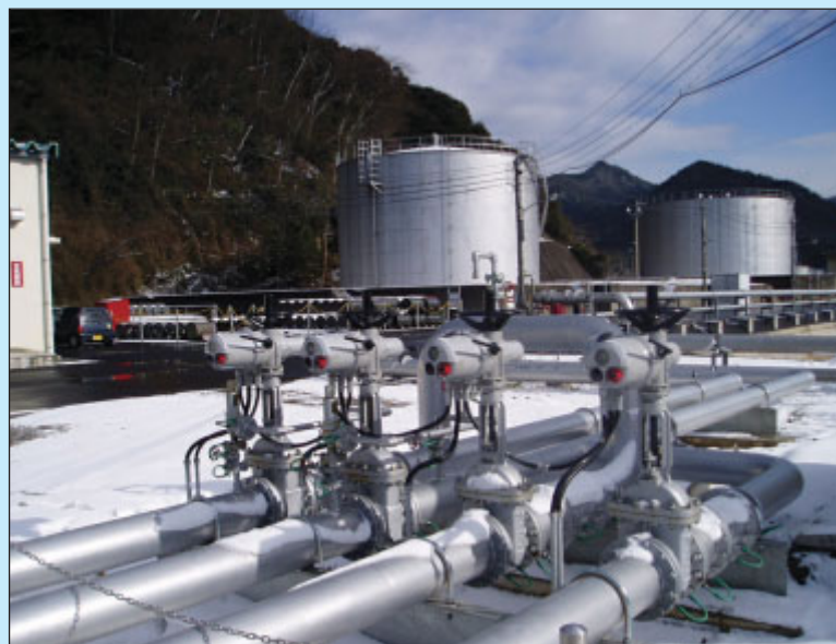
Below: Fluid System pneumatic actuator fitted to fully welded Cameron ball valve (900mm), providing gas station shut-off duty.
