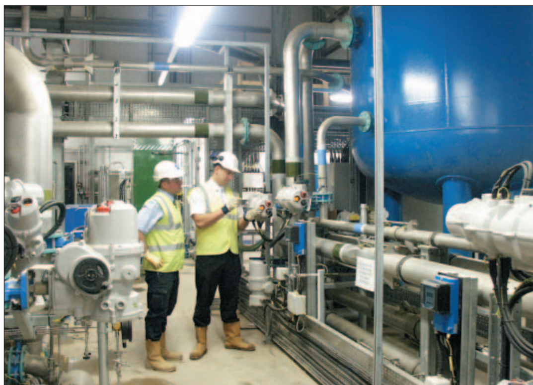
Biwater Project Manager Richard Thomson and Rotork Sales Engineer Jon Cox commissioning IQT actuators on the Pendinas filters and confirming plant status on the MCC touch screen.
