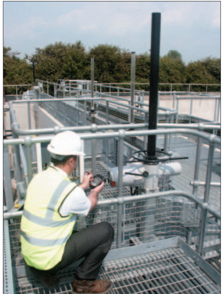
Using the non-intrusive infra red link, Rotork Sales Engineer Mike Joslin downloads operating data from an IQ actuator at Highbridge and reviews the information with Wessex Water Commissioning Engineer Iain Harris.
