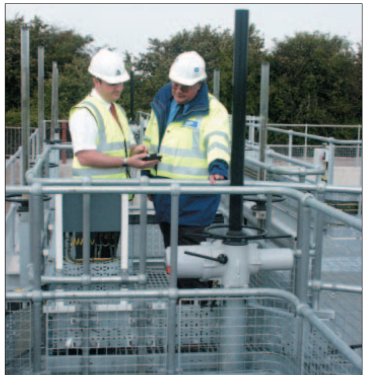
Using the non-intrusive infra red link, Rotork Sales Engineer Mike Joslin downloads operating data from an IQ actuator at Highbridge and reviews the information with Wessex Water Commissioning Engineer Iain Harris.
