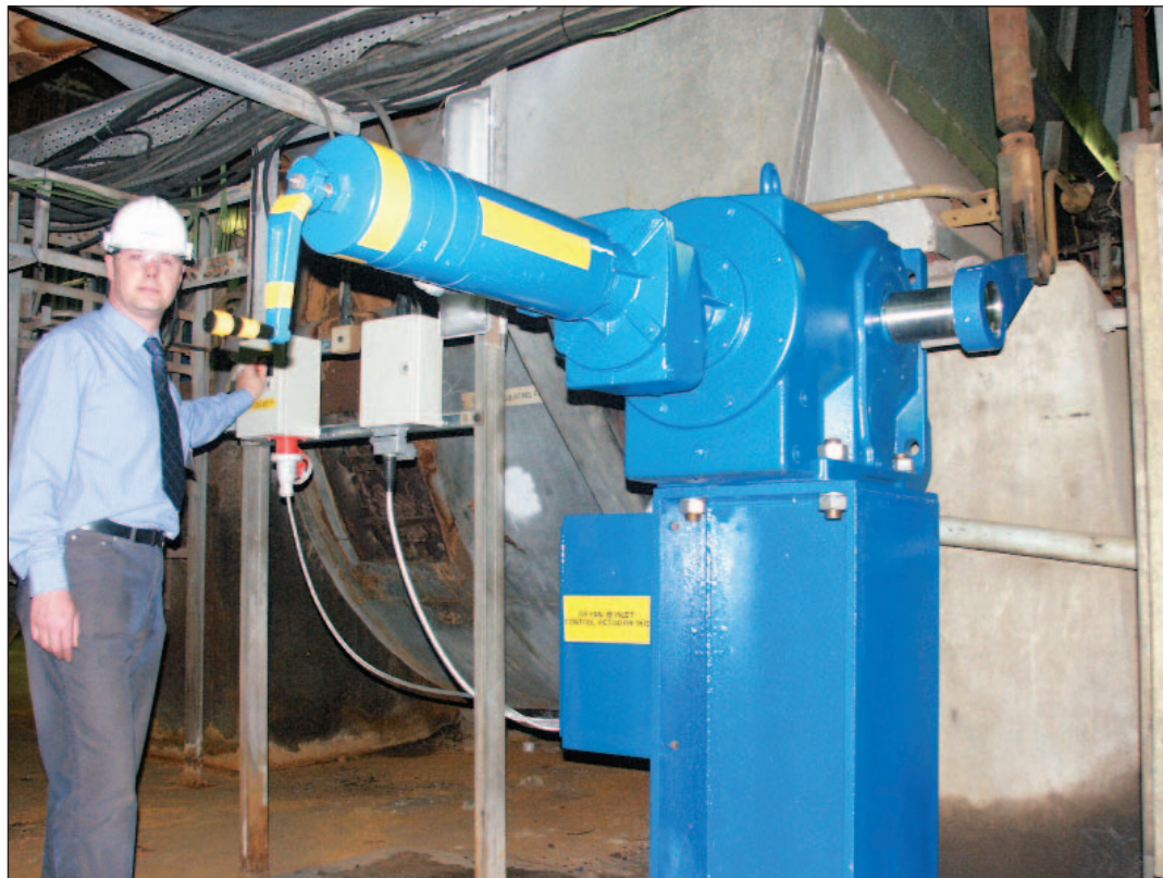
Simon Finley with the new Jordan SM6000 electric actuator installation at Littlebrook Power Station and (left) the now redundant hydraulic power pack that the actuator has superseded.
