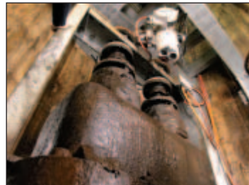
Rotork IQ actuator installation in progress on the in-situ valve.
