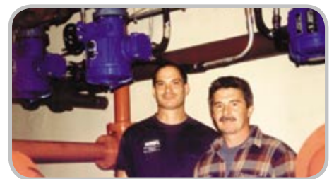
From left, Operators Timothy Pattison and John Dee stand near Rotork AQ actuators, which operate valves for the digester phase of the wastewater treatment process.
