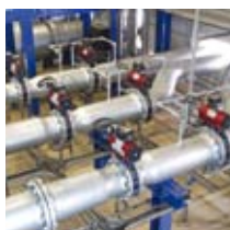
Top: RC200 pneumatic actuators at EuroLoop, the Netherlands.
