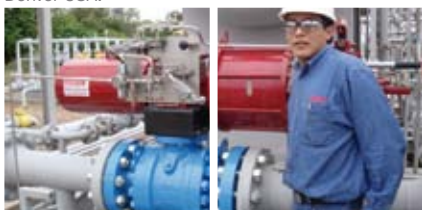
Bottom: HPG actuators on CO2 gas pipeline, Denver USA.
