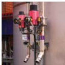
Top: RC200 pneumatic actuators, biomass power generation, Sweden.
