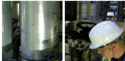
Bottom: IQT actuator on a sewage treatment aeration control valve, UK.
