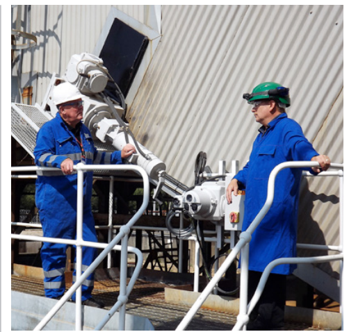
Fig 5 - Actuators on air dampers are ideal for applications where precise control and speed reduces fugitive emissions and increases boiler efficiency.
