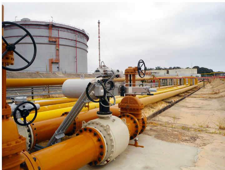
Figure 1. Rotork SI electro-hydraulic actuator operating on a pipeline.
