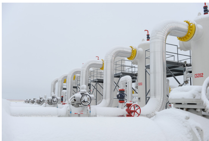
Figure 2. Rotork IQ3 actuators on a pipeline in extreme conditions.
